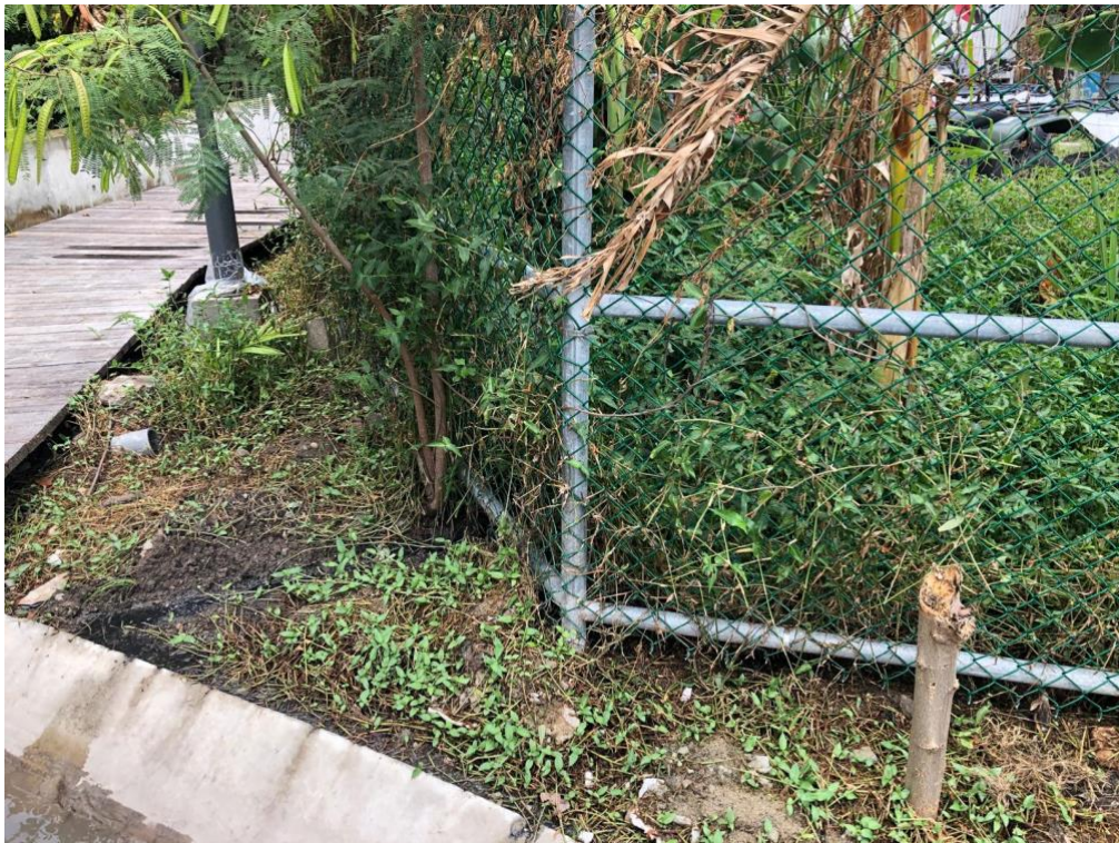
Photo 6: Evidence of overflow from wastewater holding tanks from restaurant area on Pinney's Beach adjacent to Malcolm Guishard Park
