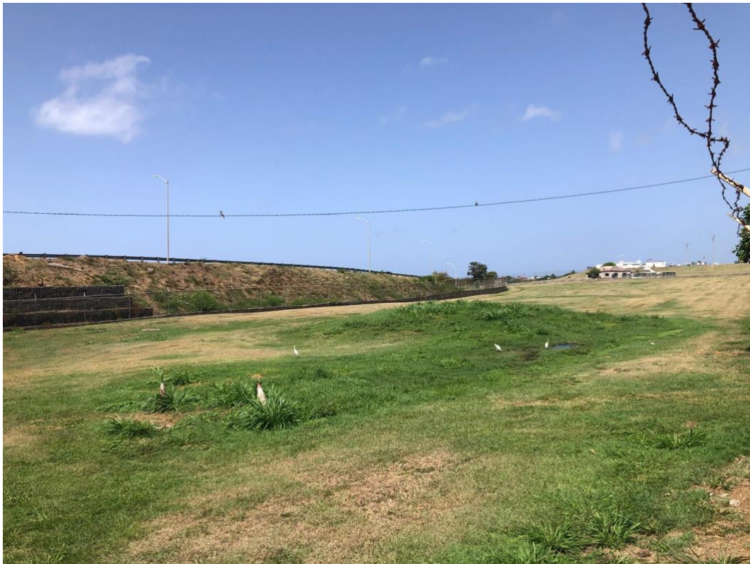
Photo 2: Stagnant water observed at leachfield of the RLB Airport treatment plant
