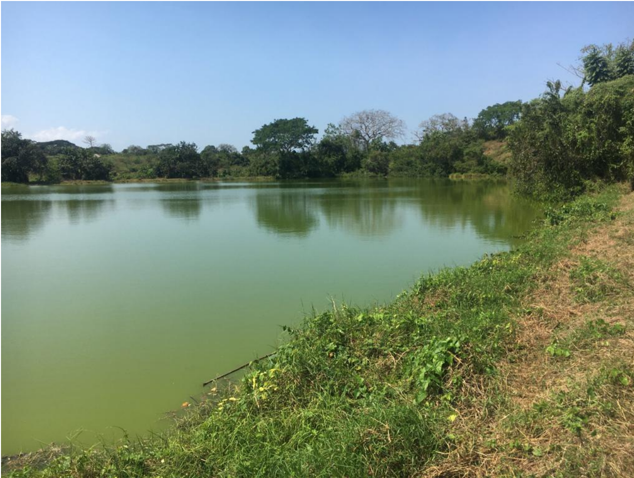
Figure: 1 Oxidation lagoon for wastewater treatment in San Antero de Córdoba, Colombia. Photo: ©GIZ/Diana García
